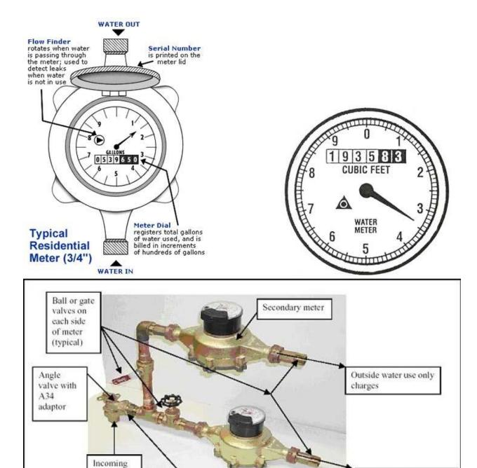
For pressure regulated areas install regulator immediately after angle valve and before tee Inside water / sewer use
